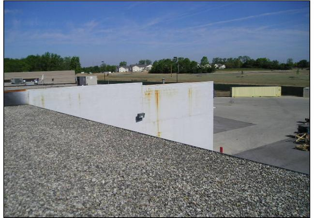
The staining on the side wall of this shopping center will necessitate the repainting of the wall. The cause of the stains is shown below.
