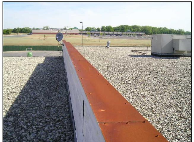
Field painted, galvanized copings will rust and if the tops are not properly treated the rust will roll over and stain the side of the building. We have even seen painters repaint stained walls and still not paint the tops of the rusted copings. It is not standard practice for painters to paint the horizontal surfaces on copings (or the outside lips of gutters). You must specifically require it or it will not normally be done. Failure to do so is almost always a mistake.
