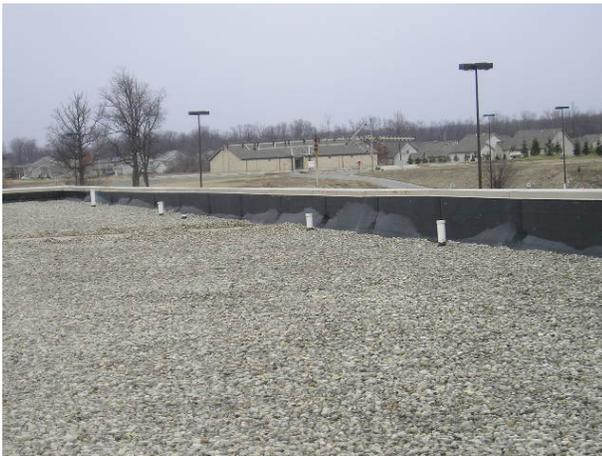
The roof shown in the picture above and in the next column is failing. The wall flashings are bridging, which is a very common failure mode for ballasted EPDM
