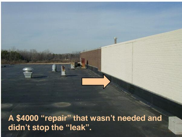
When we surveyed this roof we noted that the roof was generally in very good condition and that there was virtually nothing required in the way of repairs. But this wall flashing was brand new, clearly installed within the past few months. The cost to install it would have been about \$4000.
