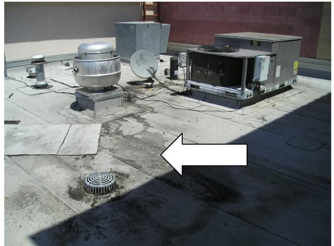
The “staining” shown in the arrow (and also clearly visible in the first photo as well) is actually a thinning of the granules because the roof has been continuously wet over prolonged periods of time. The water coming out of the P-trap should be piped all the way to the drain. This roof now needs restorative repairs which would otherwise not be required had the condensate been handled properly.
