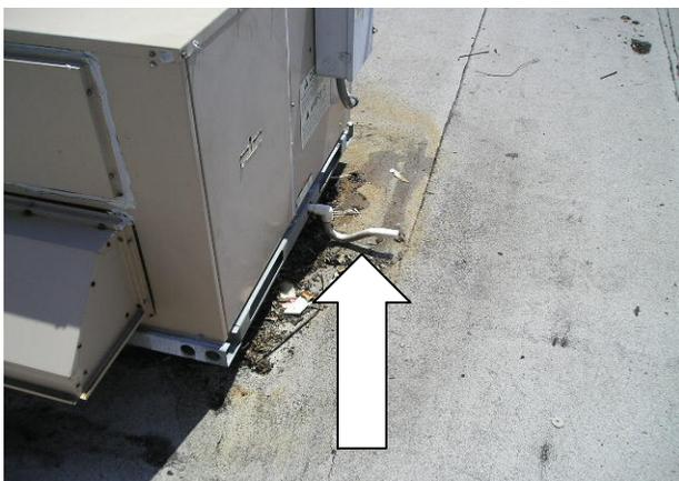
Once condensate gets out of the unit it is either dumped directly onto the roof or conducted away in piping. With built up roofs it is desirable to not dump the water directly on the roof. Continuous wetting of the built up roof surface, especially for granulated modified bitumen cap sheets and aluminized smooth surfaced roofs, accelerates the deterioration of the protective surface and shortens the life of the roof. See the next photo.
