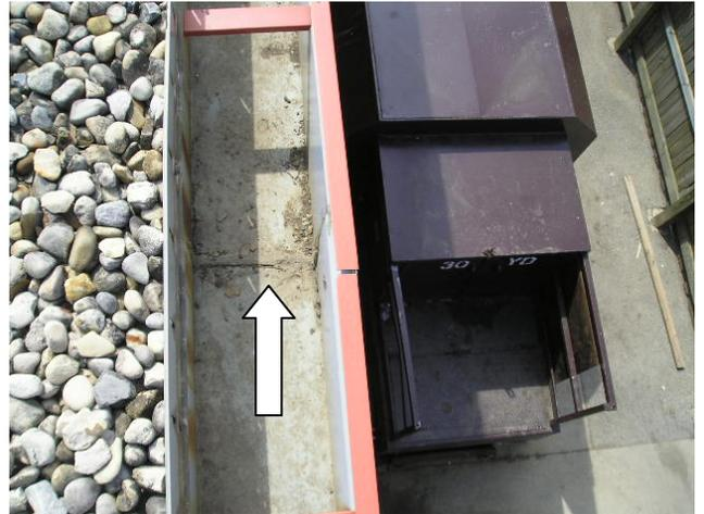
The photo above shows a typical gutter splice where sealant was applied between the adjacent pieces as the gutter was installed. This just doesn't hold up. The next photo shows a splice made with an elastomeric (rubberized) compound, specifically designed
