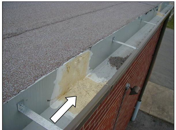
to be used in a gutter where there is often prolonged periods of standing water. Each splice is reinforced with a piece of mesh embedded in the coating. So, as the gutter moves the splice can flex with it. This is the right way to seal a gutter and is much cheaper to do in the long run.
