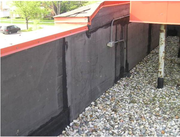
One of the most common problems on older EPDM roofs is a phenomenon known as “bridging”. The top photo shows what a properly functioning wall flashing should look like. The material is tucked neatly into the corner at the junction between the horizontal surface of the field of the roof and the vertical surface of the parapet wall.
